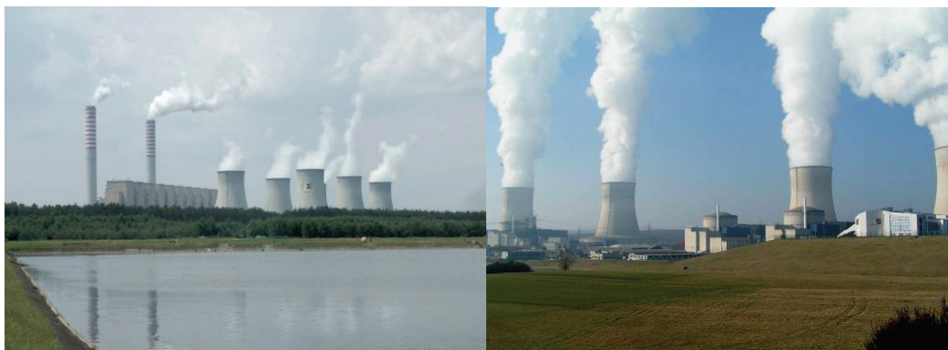
Figure 8. Coal and nuclear power plants
