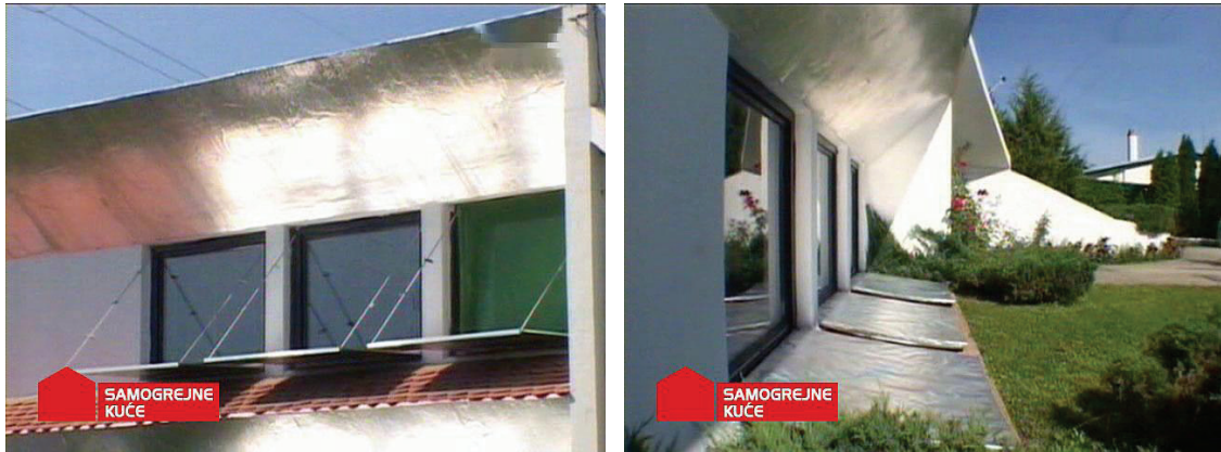
Figure 2. Reflective panels – the third decade of their use. As it can be seen in the photos, the bottom panels are movable.
